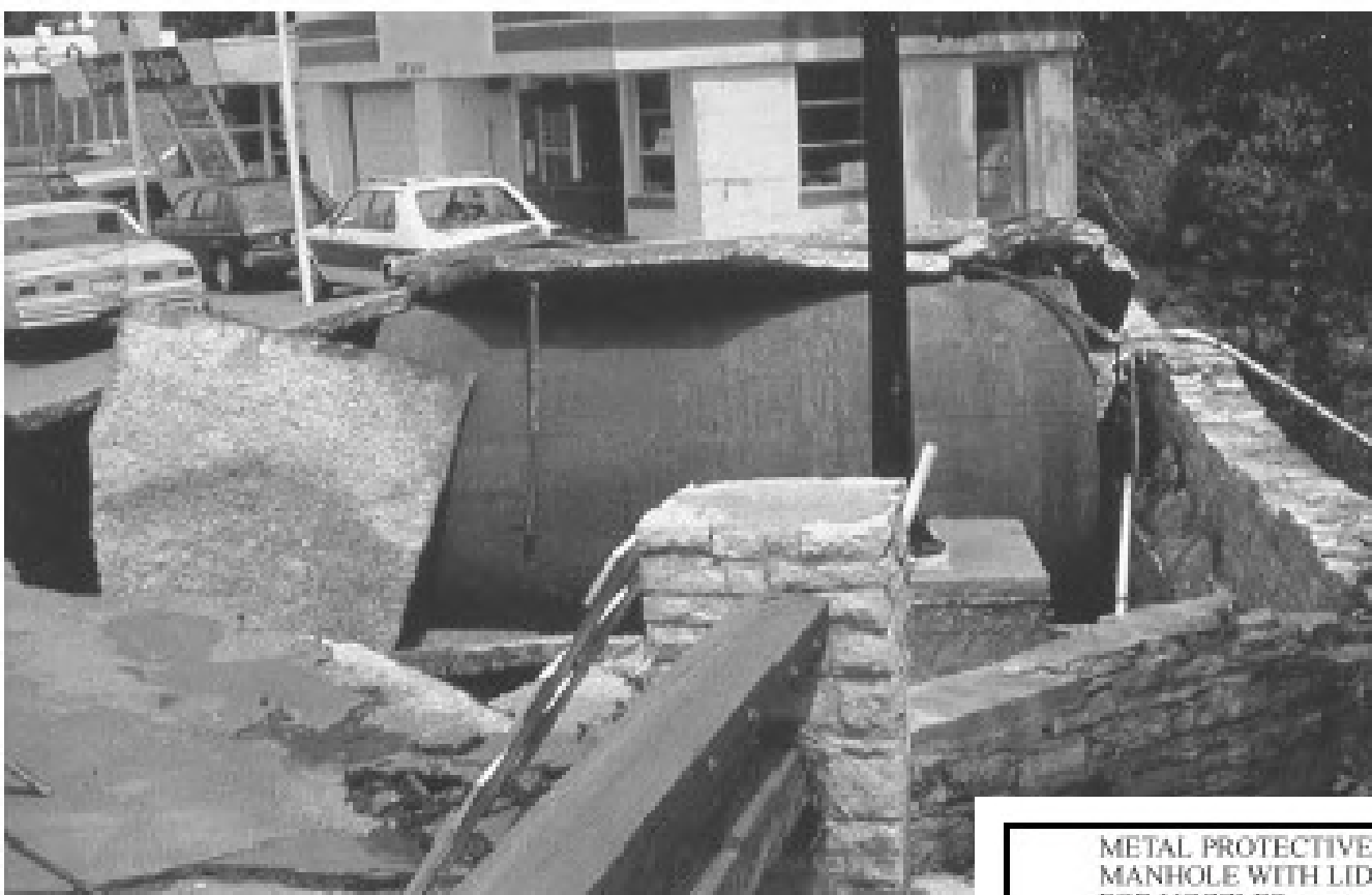
Figure 3.2.3.1A: Tank lifted by buoyancy forces
