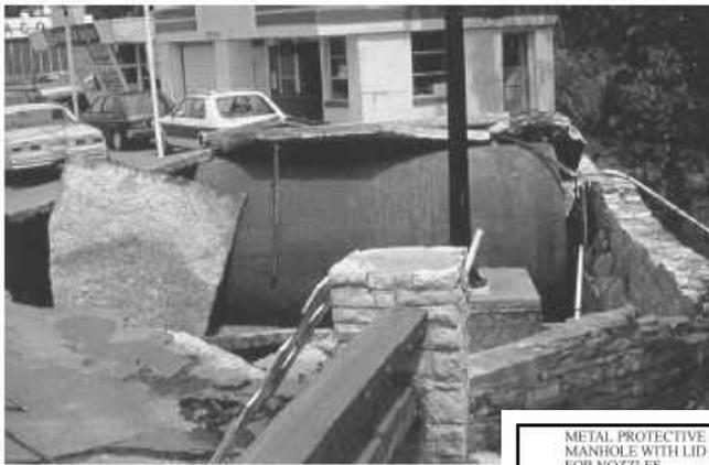
Figure 3.2.3.1A: Tank lifted by buoyancy forces
