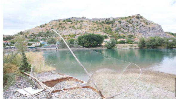
Iron boxes filled with gravel for flood defence are 6 mt higher than the normal river level.
